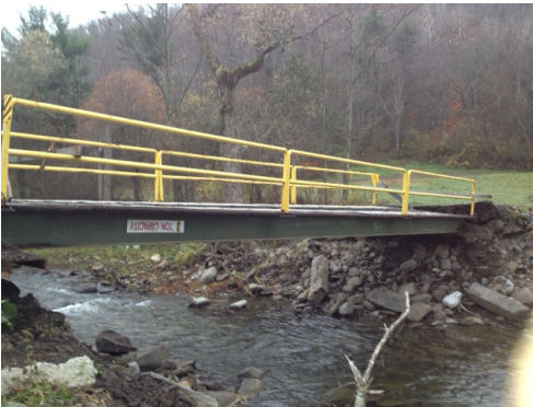
The Mann bridge by the Maple Inn was closed after the embankment was eroded by storm waters.
