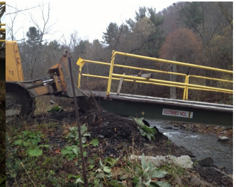
To prevent the bridge from washing away during the coming hurricane, dozer operator Karl pull the bridge to safety.
